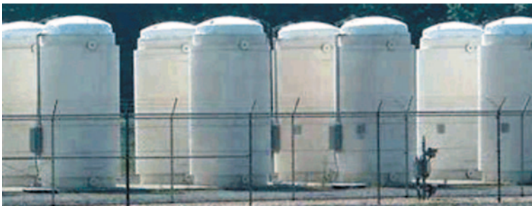
Fig. 21.2 Nuclear waste disposal container. (Source NEI)
