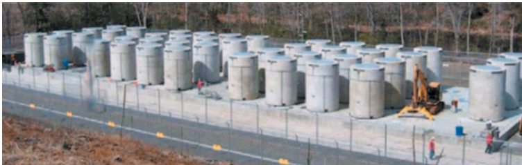
Fig. 19.4 During temporary storage, the radioactivity and heat of spent nuclear fuel decreases significantly
